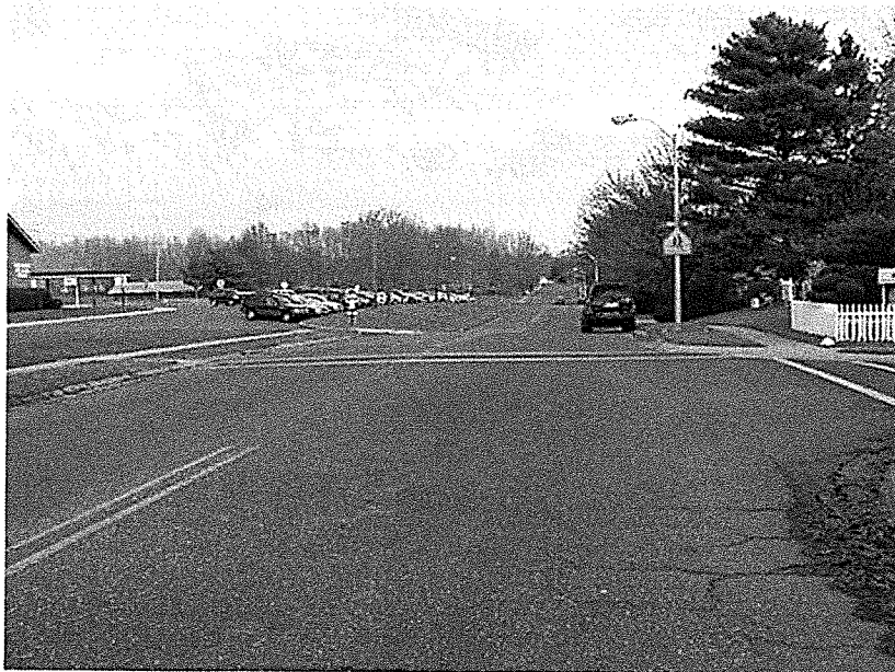
Intersection of Evergreen Drive and Ember Lane (Northside)
